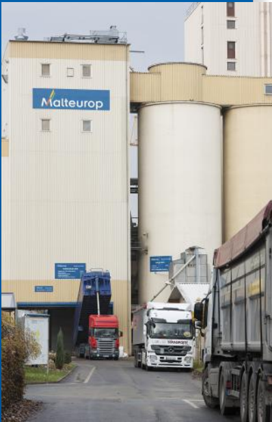
The European malt producer Malteurop uses Guntner air heater coils as well as thermowave plate heat exchangers in its refrigerating plant.
