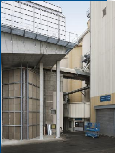
Ten Guntner GCO air heater coils (still without casing in the image) produce hot air for the kiln.
