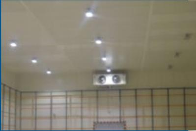
▲ An LT cold room for 1,000 metric tons/1,102 short tons cooled by two Güntner CUBIC Vario CPGHN evaporators mounted at both ends of the room, blowing face to face.
