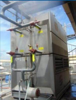
▲ Two Güntner ECOSS evaporative condensers dissipate the waste heat of the NH<sub>3</sub> compressors into the ambient air.
