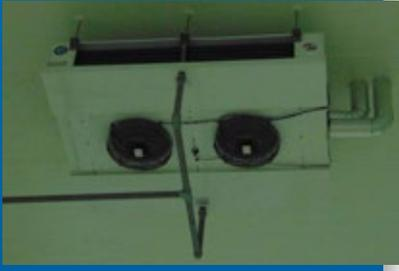
▲ Güntner DUAL Vario air coolers, type CPDHN, provide the required cold for the anterooms.
