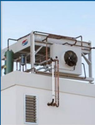
▲ A Güntner condenser FLAT Compact GVHX with separate Güntner subcooler VERTICAL Compact GSVC with microox technology on the roof of the machine room.
