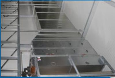
▲ Two floor-mounted Güntner brine air coolers FLOOR, type GSN, transfer cold to the hop storage that is kept at a constant 2 °C/35.6 °F.
