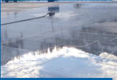
▲ There is an efficient aluminium pipe system in the tray under the ice surface to freeze the water to the required temperature and consistency, and to maintain the temperature of the existing ice.
