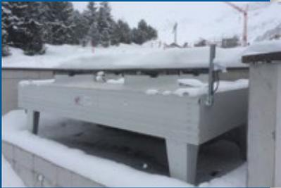
▲ A Güntner FLAT Vario GCHV condenser dissipates the heat from the primary cooling circuit to the environment.
