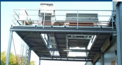
Condensers mounted on a steel construction next to the machine room.
