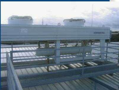
A Gntner S-GVH condenser with subcooler on the roof of the machine room
