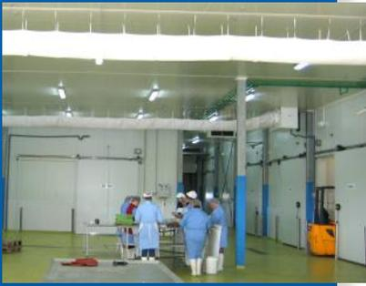
The cold air streams from the cubic Gntner GHN air coolers into the work areas through textile socks.
