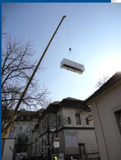
A crane lifts the fluid coolers on to the roof of the ICU IPS1.
