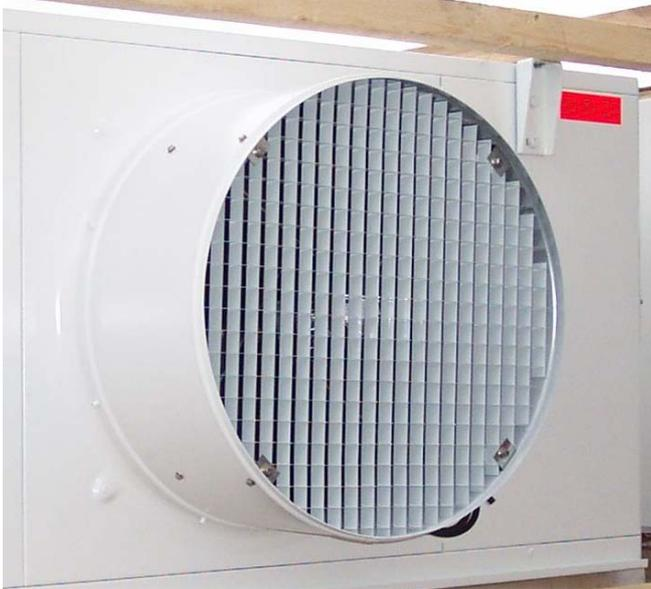
Figure 6: Air rectifier grid
